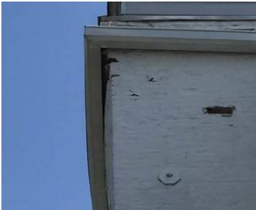
structure. The inspection also determined that, over time, the bell tower has started to pull away from the back of the church building. The structure has shifted significant enough that it has created a fall hazard from above. Until we can investigate further, a temporary tunnel of scaffolding has been put in place to protect from the potential hazard of falling
